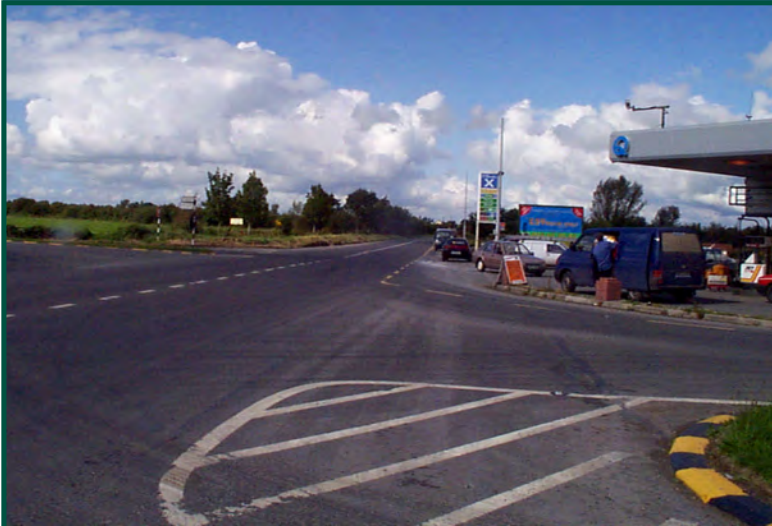
Before road safety remedial measure implemented
