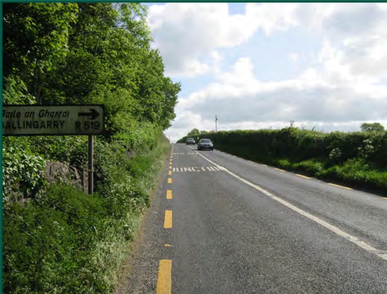
Before road safety remedial measure implemented
