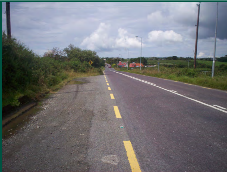
After road safety remedial measure implemented
