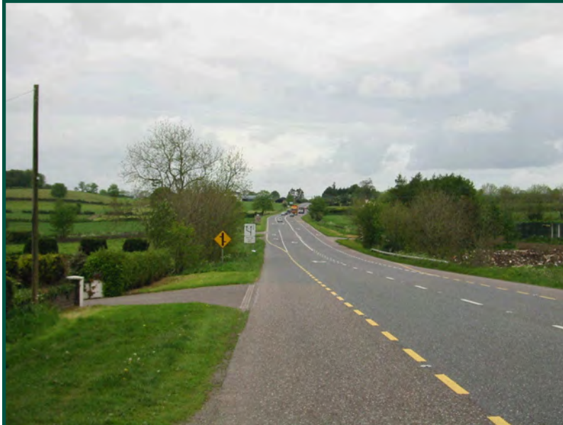
Before road safety remedial measure implemented
