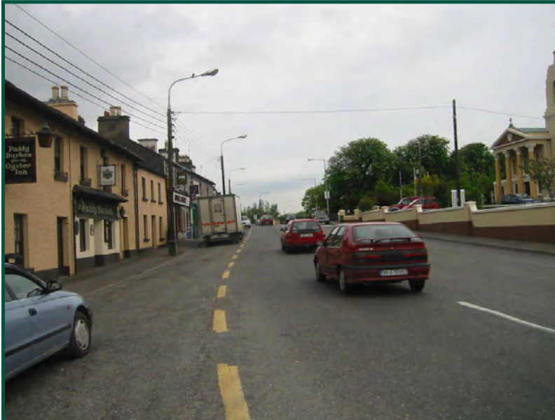
Before road safety remedial measure implemented
