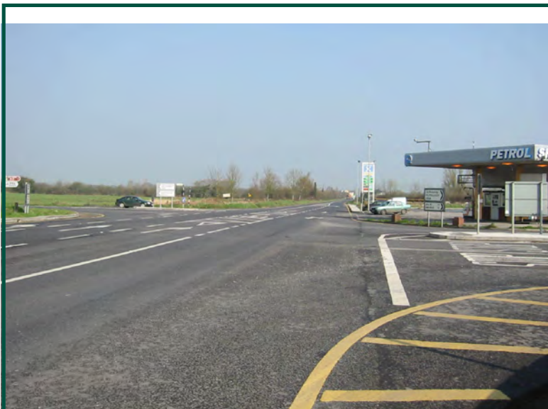
After road safety remedial measure implemented
