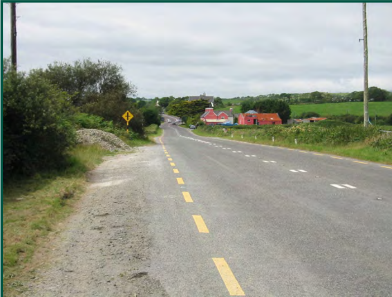
Before road safety remedial measure implemented
