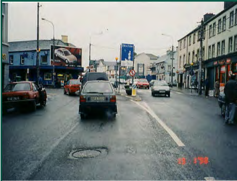
Before road safety remedial measure implemented
