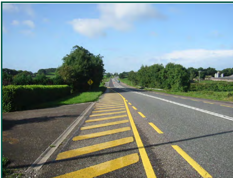
After road safety remedial measure implemented
