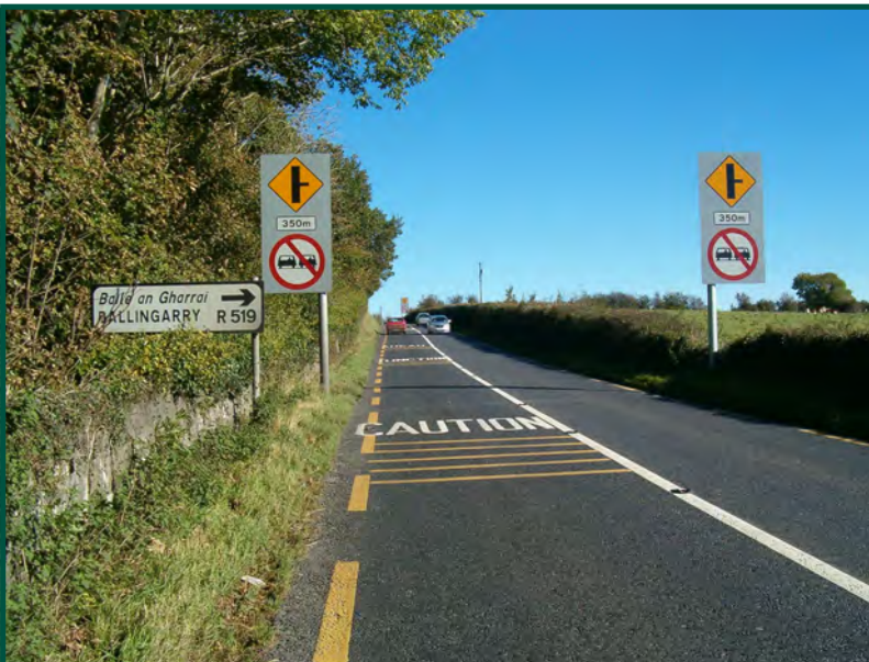
After road safety remedial measure implemented
